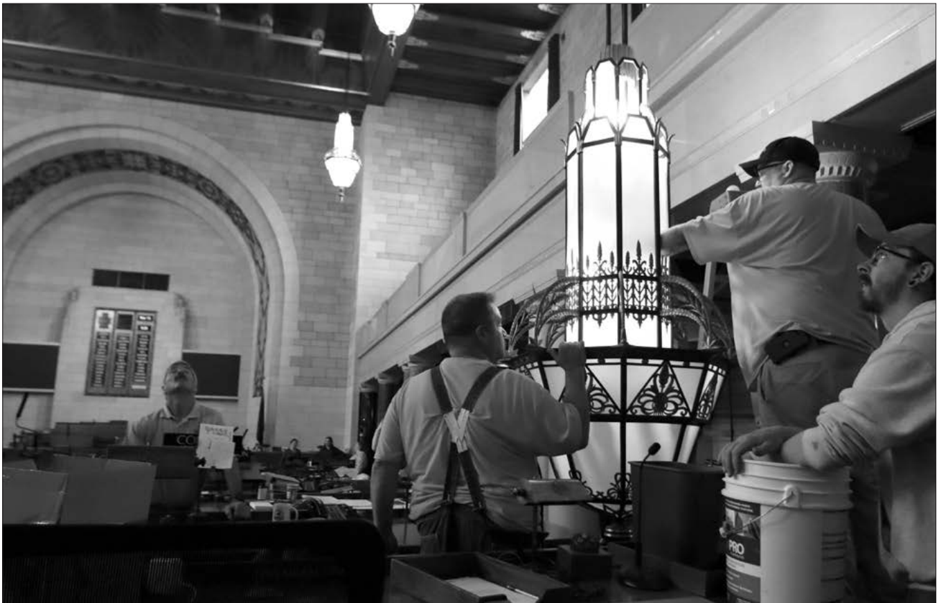
Office of the Capitol Commission employees lowered chandeliers in the George W. Norris Legislative Chamber March 13 to replace light bulbs.
