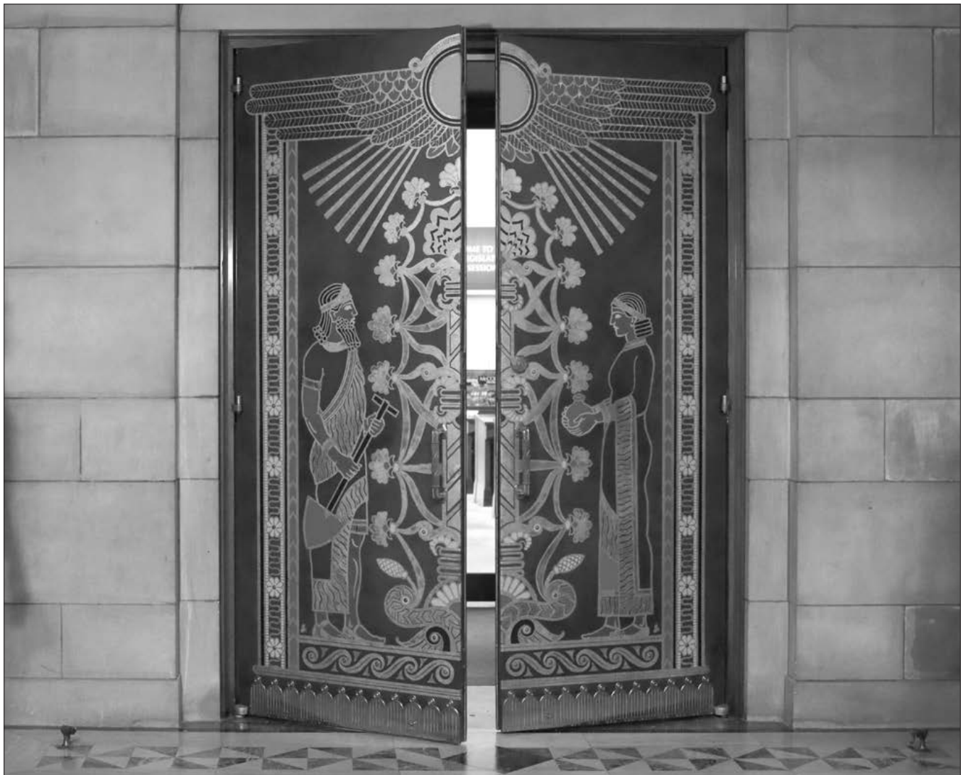
The doors of the George W. Norris Legislative Chamber were reinstalled Jan. 6, after a year of work to reproduce the hand-tooled, hand-painted leather covering and restore the wooden door structure. The original leather had become dried and cracked since its original installation in the 1920s.
