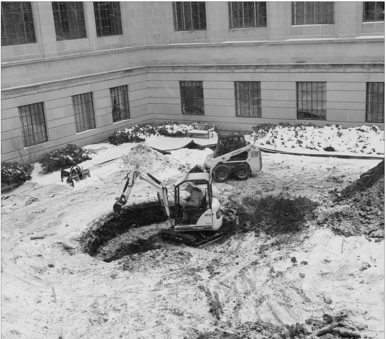
Construction crews continue preparations for new fountains in the Capitol courtyards.
